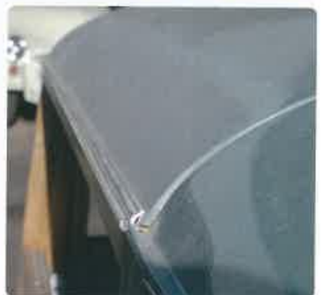
11 As well as meeting neatly above the rear doors, the mouldings need to be aligned with the drip rail on the front bodywork section.
